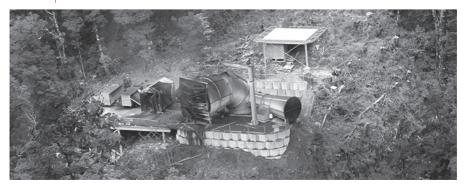
The blackened ventilation shaft at the Pike River mine, damaged by the earlier explosion - November 2010.
